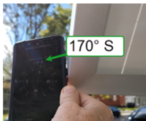
Figure 11, Aiming the panel to Solar South with a compass app
